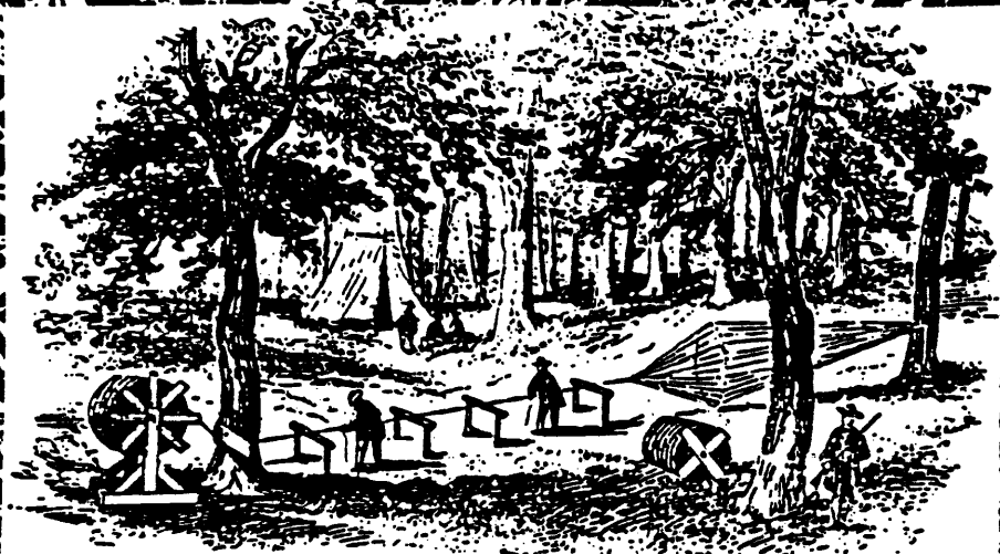
Cable for a river crossing was spun on the spot. Submarine cables were used later when gutta percha proved to be a good underwater insulator.
