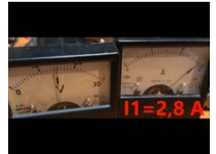
Measuring the total amperage of the circuit: I1.
