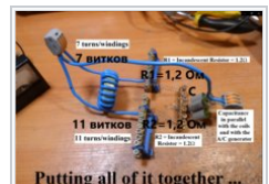
Building the circuit to test a shorted transformer. ↗
