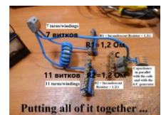
Building the circuit to test a shorted transformer.
