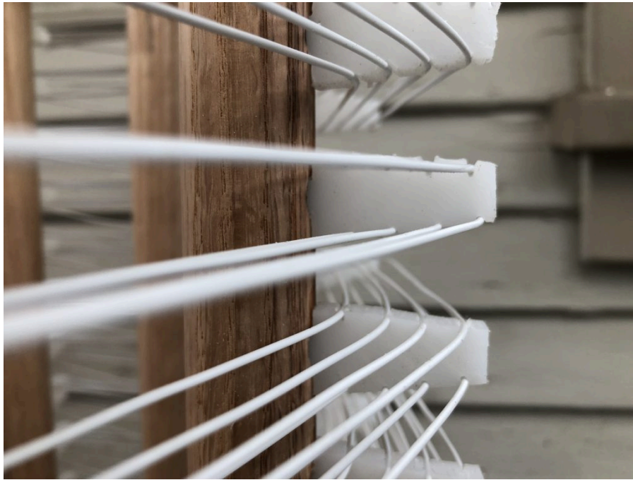
Fig. 7. – Close inspection of the insulator supports.
